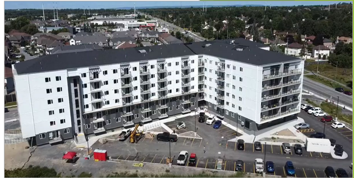
Eagle Point ( 800 Eagleson Road. Kanata ) – Completed
